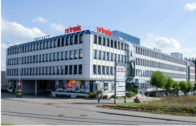
Rotronic Headoffice (Bassersdorf, Switzerland)
